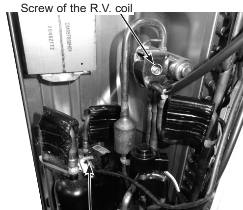
Discharge temperature thermistor
