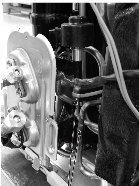
Brazed parts of LEV valve
