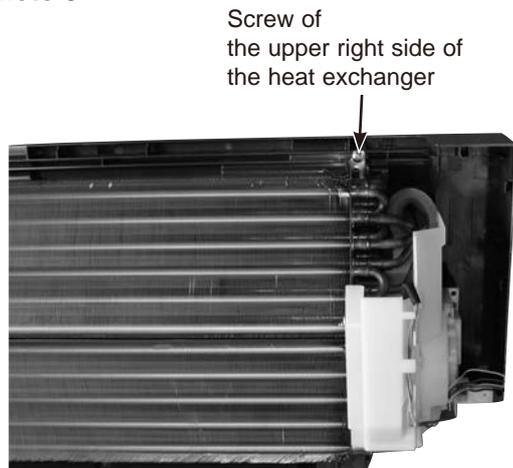
Screw of the upper right side of the heat exchanger
